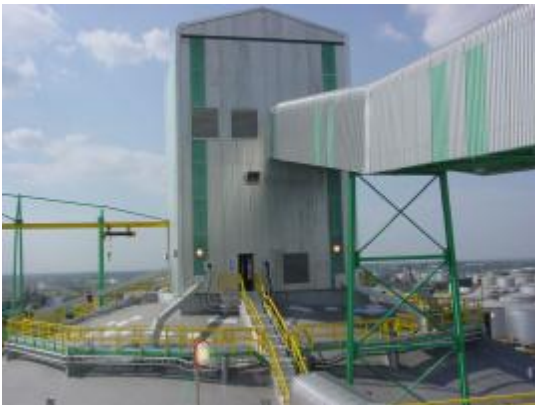
Alumina Feed Conveyor Steel Structure
